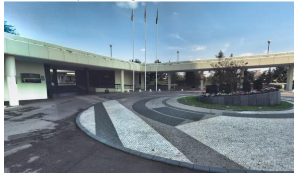
Location B Lower level, view from SE
