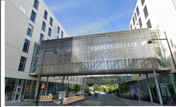
Bridges between buildings are placed in the field of view of the competitor → canopy.
