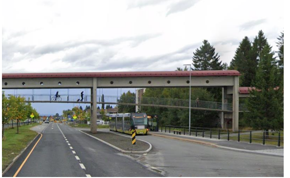
Canopy over the bridge (possible to pass under) → canopy can be omitted, two-levels are mapped
